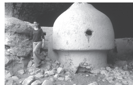
Detail of Granary - Exterior 4" bench inset and ventilation shaft
